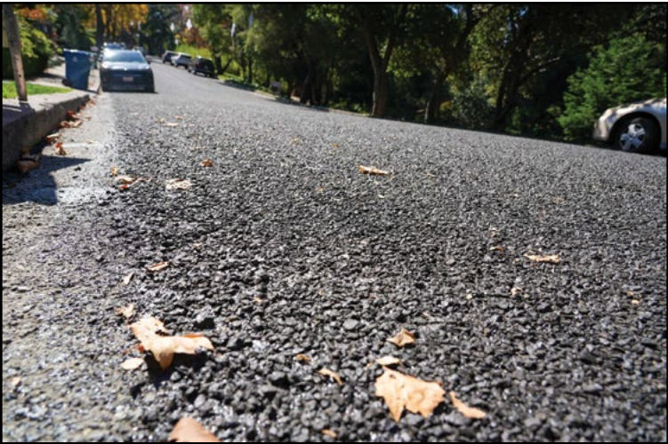
Photo by City of Piedmont Dracena Avenue's repaving received the "chip seal" fix.
